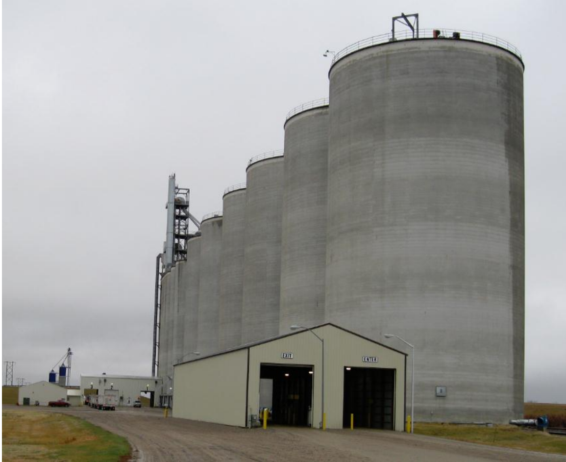
Image 2. Alton Grain Terminal, truck weighing and dumping; 3 dump pits with 45 trucks/hour capacity
